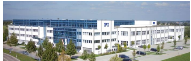
PI headquarters in Karlsruhe, Germany: More than 350 employees work on high-resolution drive systems and positioning systems
